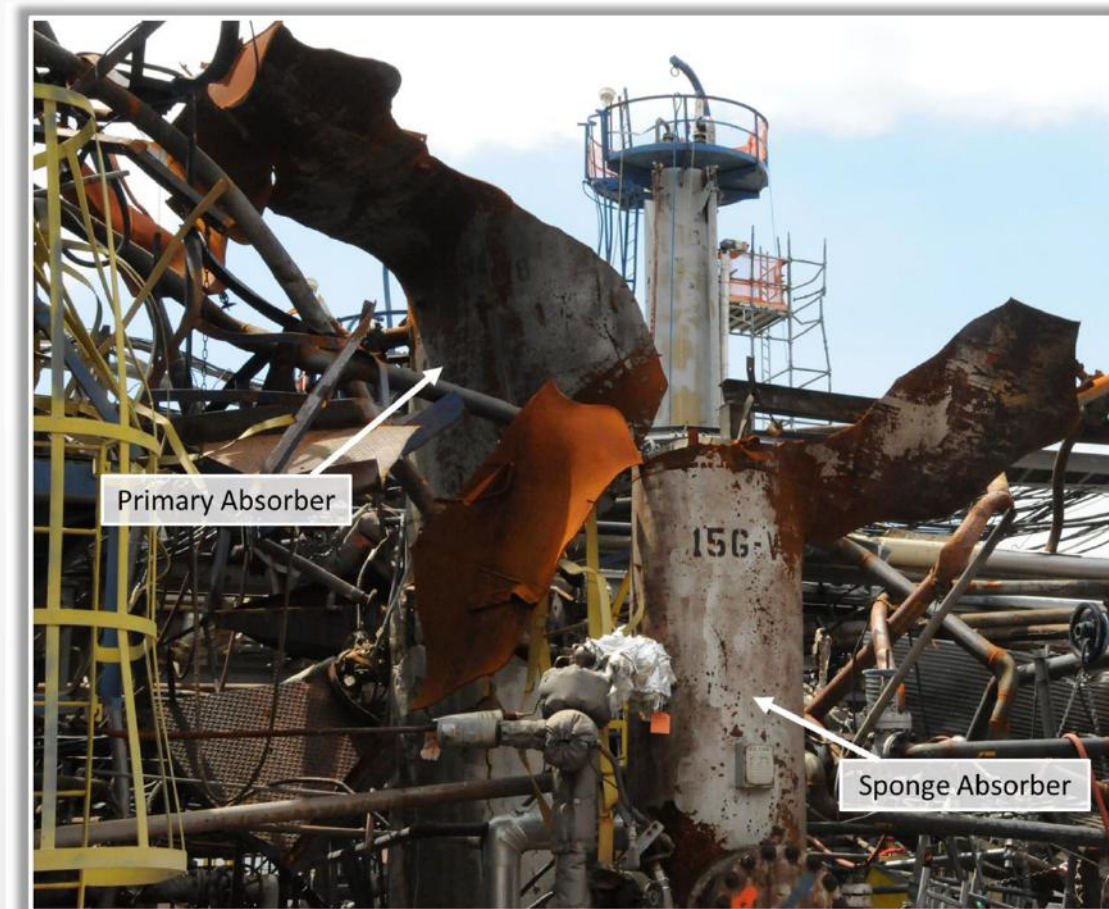
Figure 45. Primary and sponge absorbers after the incident. (Credit: CSB)
