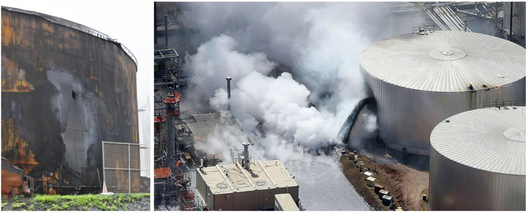
Figure 18. Asphalt tank puncture and leak. (Credit: CSB [left], Duluth News Tribune [right])
