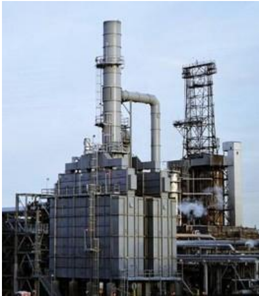
Example of Delayed coker furnace
