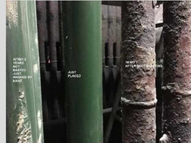
TP310H outer coated tube before boiler cleaning [plant stoppage] (after 2 year service)
