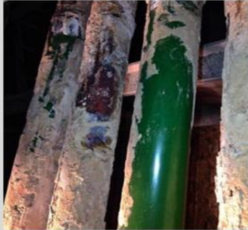
TP310H outer coated tube before boiler cleaning [plant stoppage] (after 1 year service)
