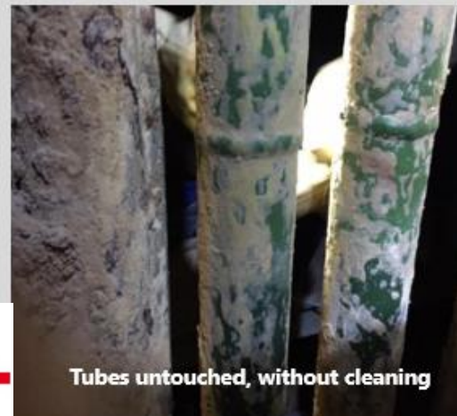
TP310H outer coated tube before boiler cleaning [plant stoppage] (after 2 year service)
