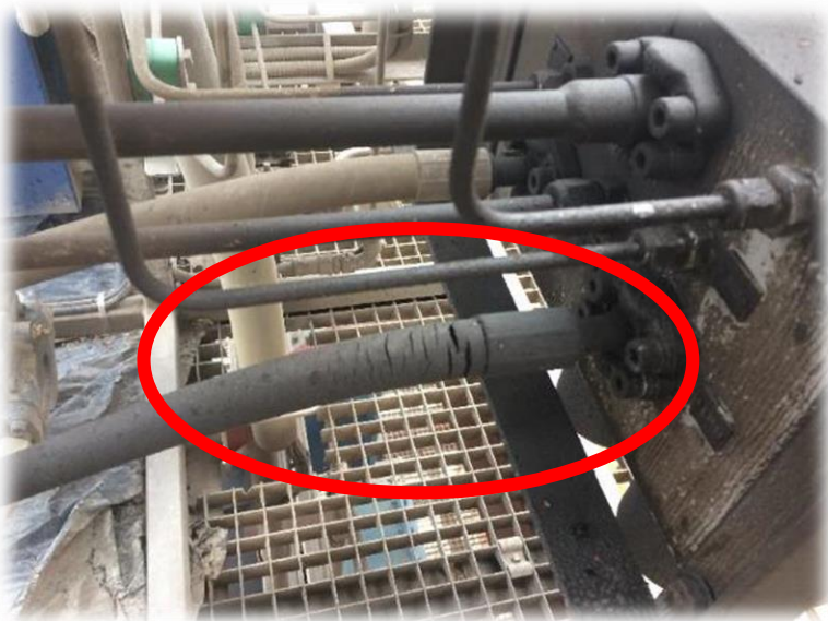
Defective / Worn Out of HPCU Equipment & Hoses/Pipes
