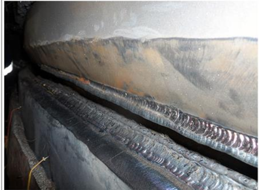
Reconstructed Bevel Ready for Root Pass
