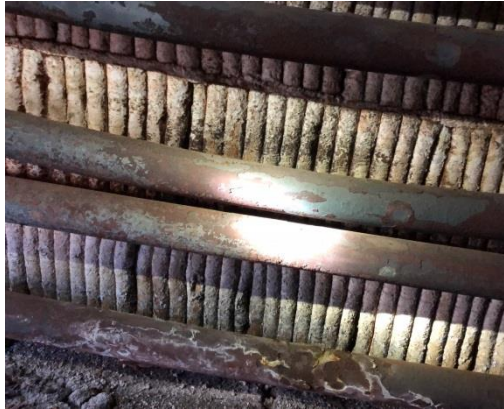
Side wall radiant tubes
