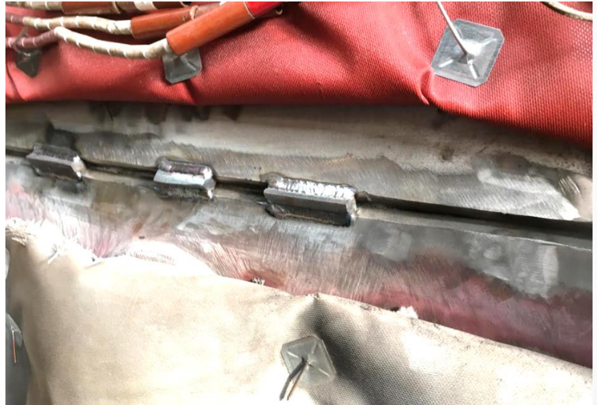
Proper Root Opening for Welding
