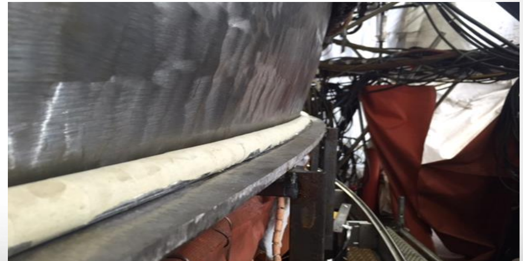
STEP 3. INSTALL WELD BACKING
