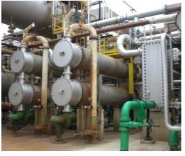
Pos 12: Compressor interstage condensers, WPHE = 5,1 MW, start-up 2009
