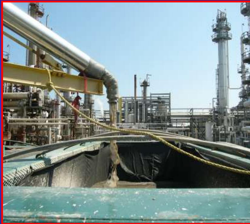
Clarifier Underflow Dumping to Settling Bin
