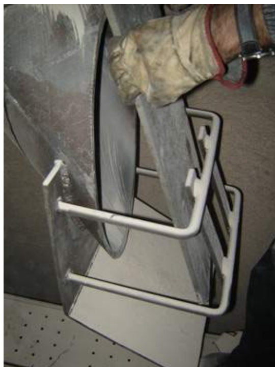
Figure 6 – Cyclone Dipleg Check Valve
