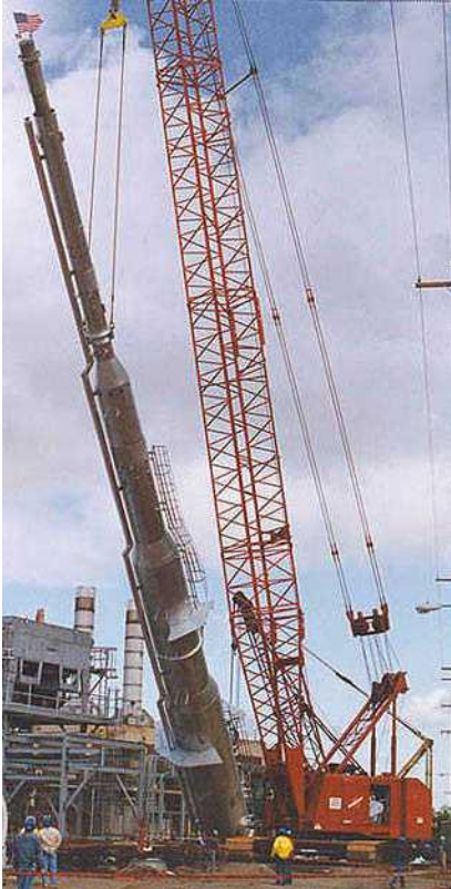
Figure 4. Tail gas incinerator with a flare
