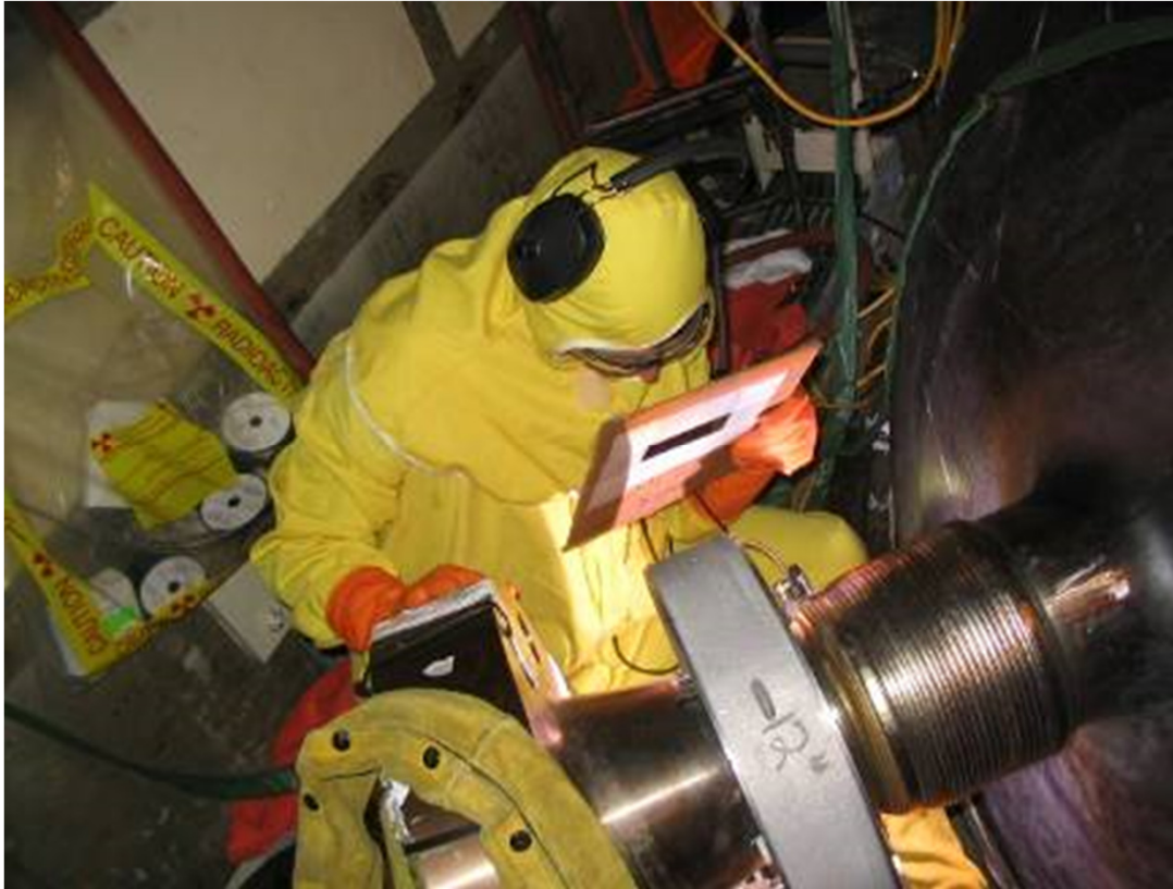
Small nozzle structural overlay in pressurizer vessel
