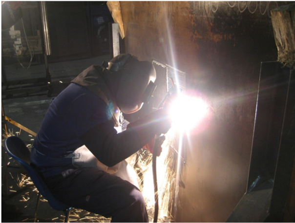
Removal of bonded cladding
