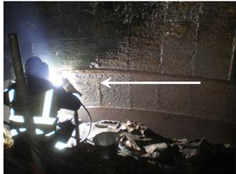
Gouging in process 2 – 3 mm material removed
