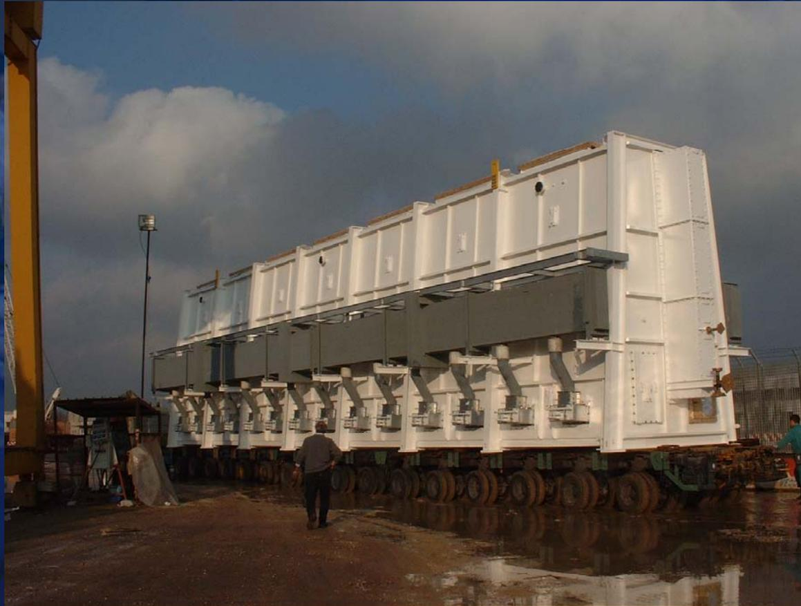
**Radiant Cell Fully Assembled**
