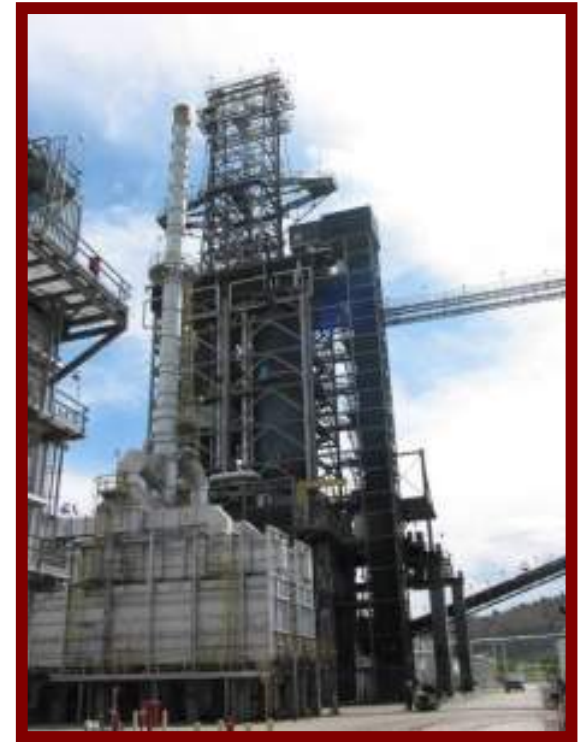
Billings Refinery Coker Courtesy of CoP
