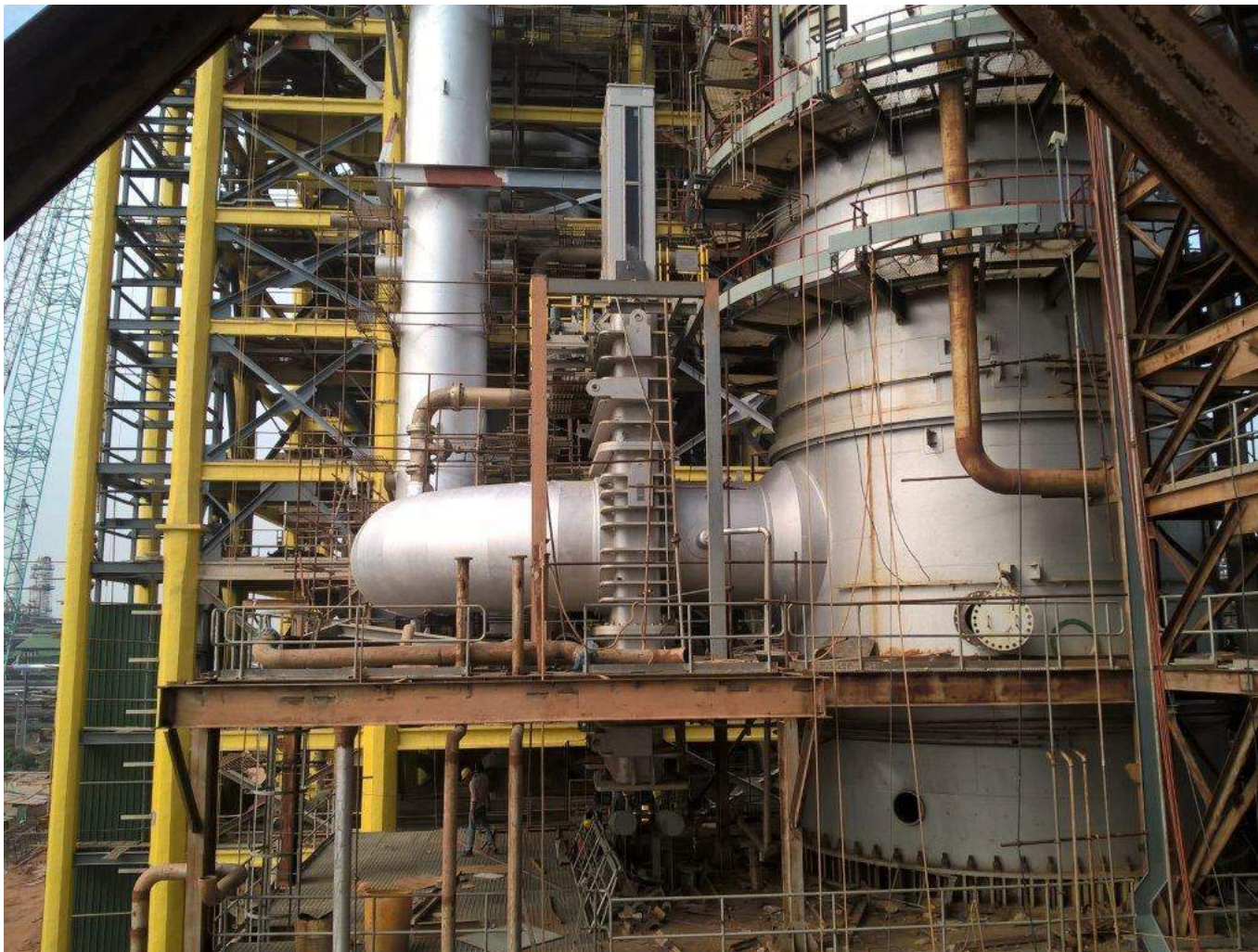
100" FCC Reactor Overhead Line Valve Installation
