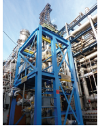
Test unit in place
