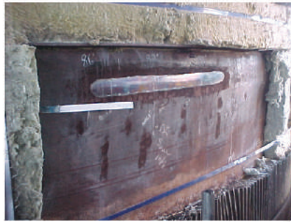
Inco weld repair from O.D. surface.
