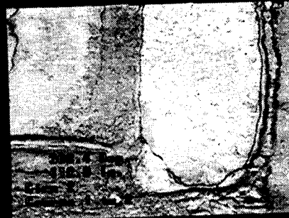
Crack in overlay
