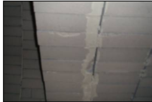
Figure 9. Displaced Bullnose Brick
