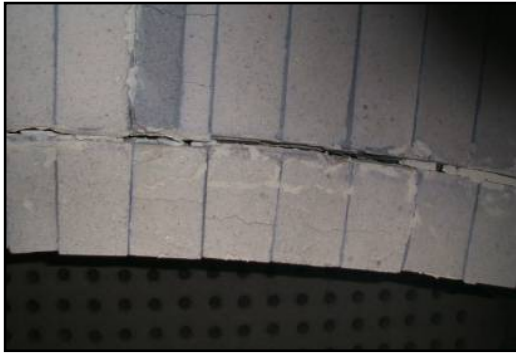
Figure 8. Bullnose Brick Sag
