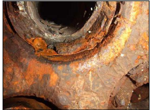
Figure 12. WHB Tubesheet Joint After One Year of Service (From a non-Ortloff licensed unit, not one of the case history SRUs)
