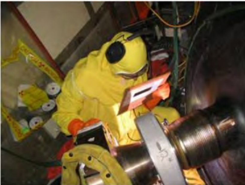
Welded Structural Overlay Being Applied
