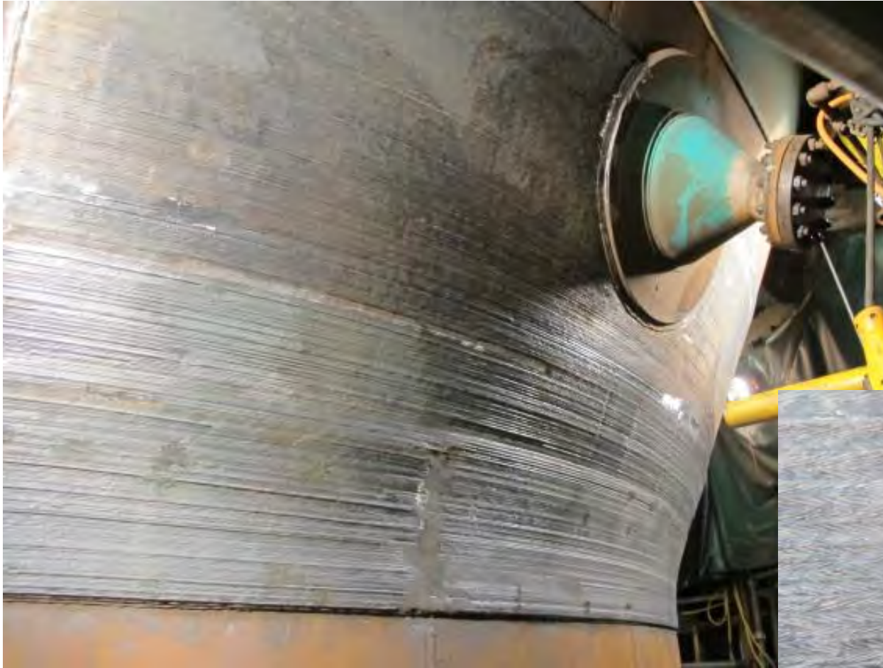
Finished Structural Overlay (three layers)
