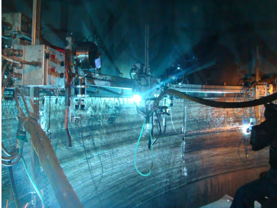
Typical bulge overlay repairs inside of the coke drum
