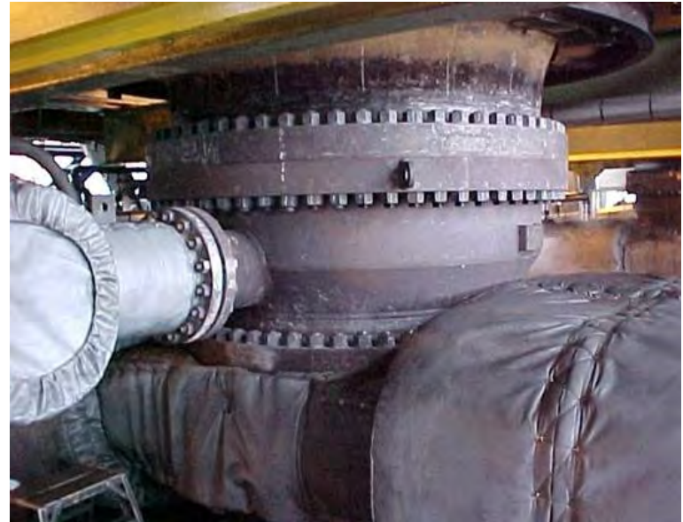
Enclosed Slide Valve Bottom Unheading System
