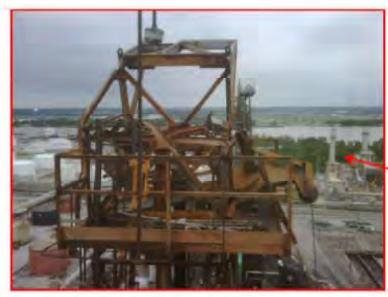
In addition to the "A" drum, "B" drum was rendered inoperable since the two drums share a common bottom unheading system. The "A" bottom head was un-headed at the time of the derrick failure. Sunday May 9, at approx 9:00 AM the top 8-10 feet of the Far East Coker derrick collapsed while cutting a drum and attempting to free a stuck drill stem.
