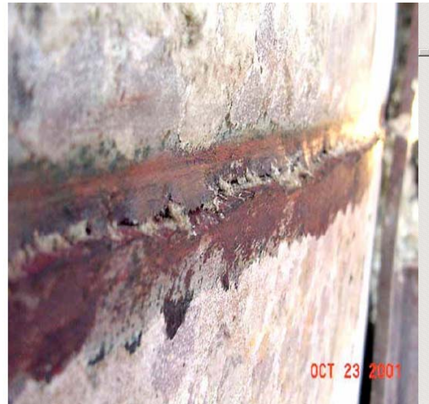
Typical Skirt Cracking
