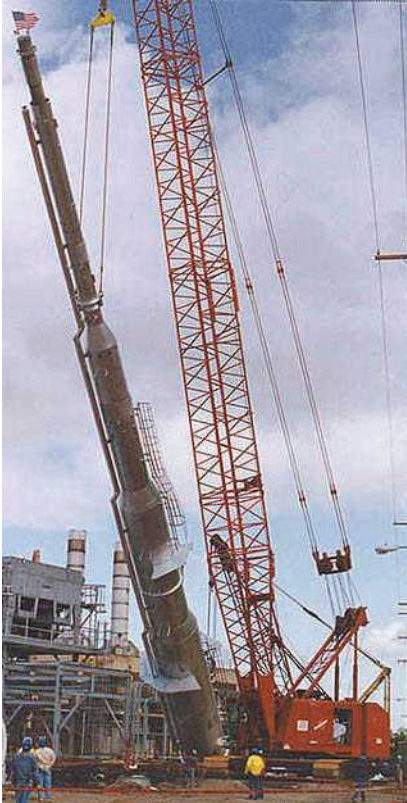
Figure 4. Tail gas incinerator with a flare
