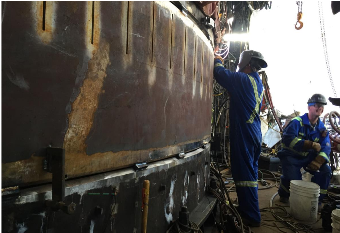
Final Fit-Up after Tacking
