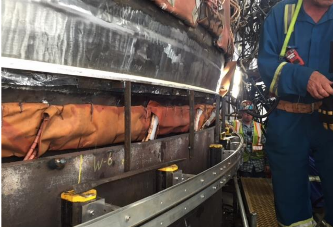
Casting Insert (White) and Welding Shelf
