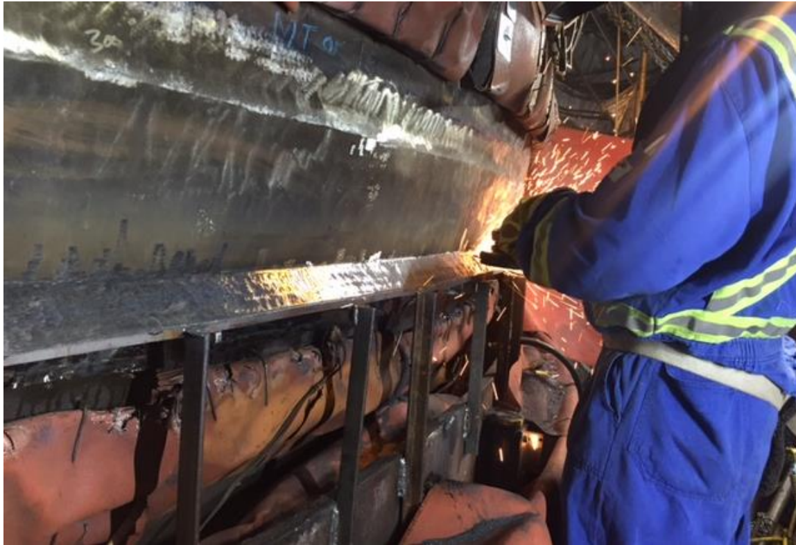
Surface Shaping of Deposited Knuckle Weld
