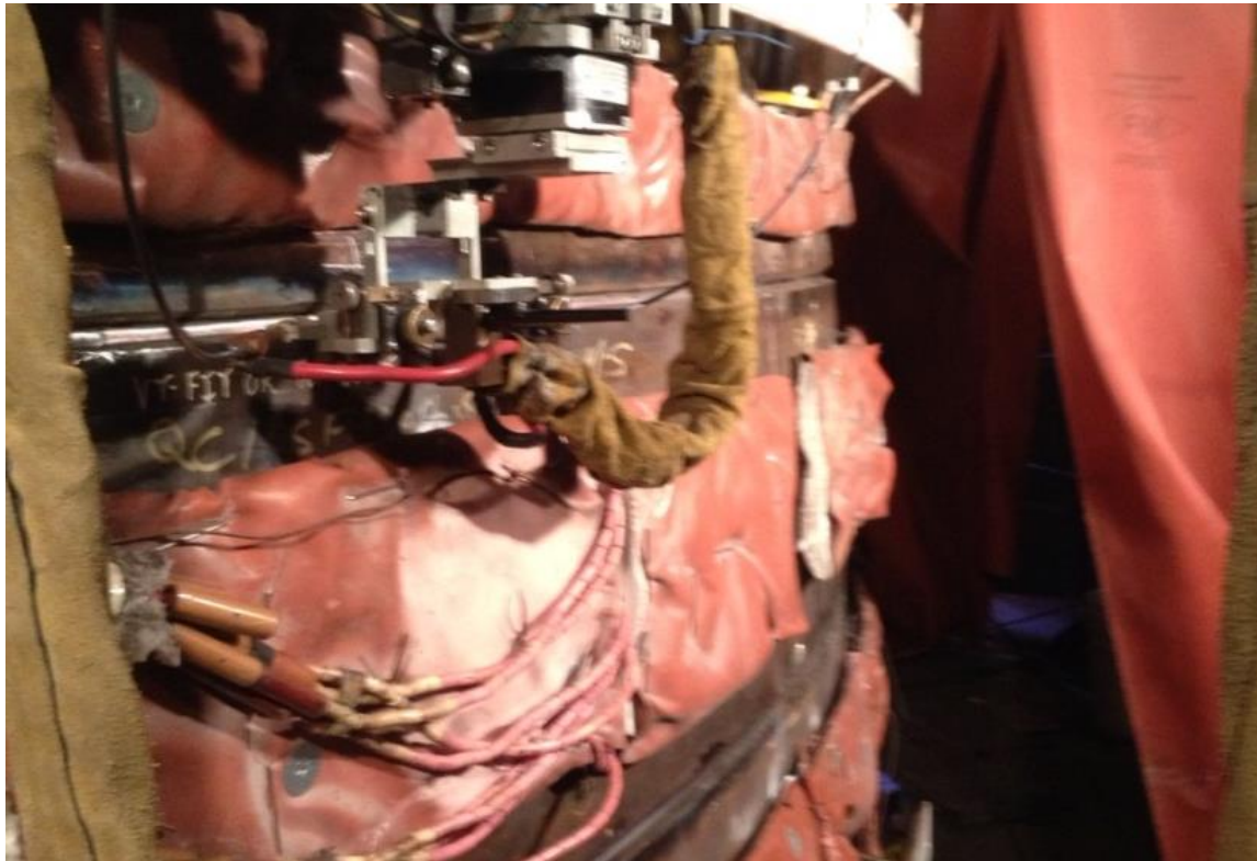
GTAW Hot Pulse Welding System Installed
