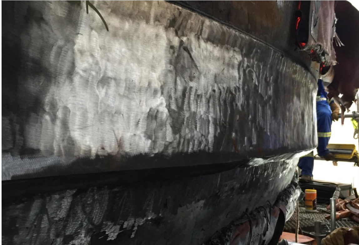
Front Surface of Knuckle Weld Deposit (After Blending and Surface Profiling)
