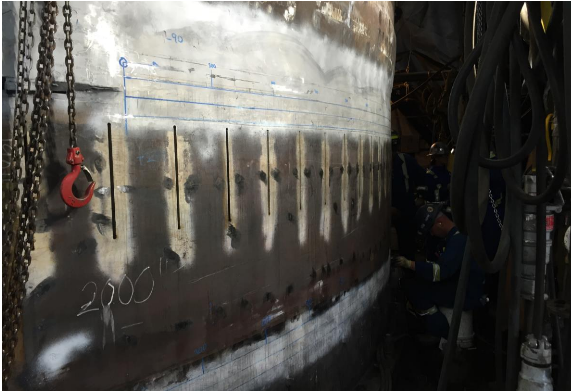
Final Appearance after Installation (Inspection: Liquid Penetrant Inspection and Linear Phased Array)
