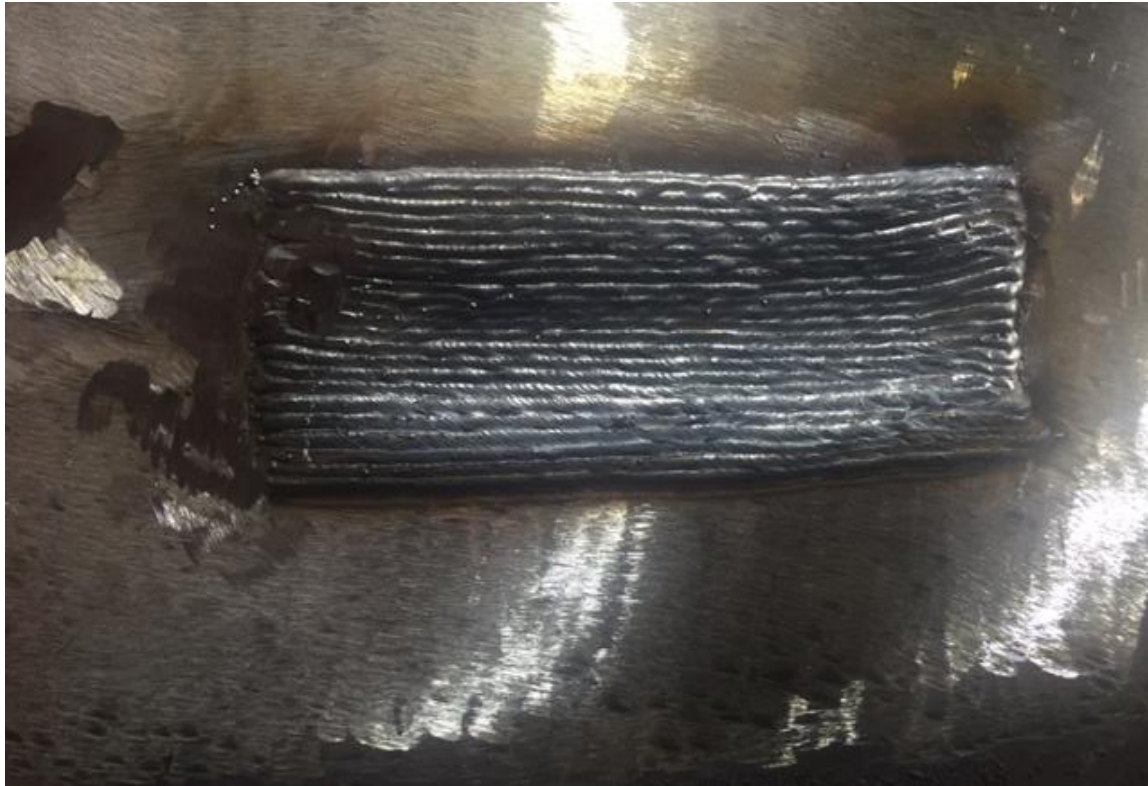
Repair Welding of Cone Base Material (2 Layers Required to Achieve Tempering)
