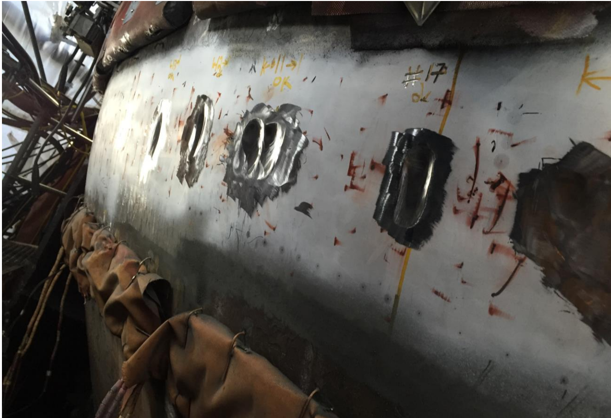
Removal of Flaws Detected with Magnetic Particle and LPAUT
