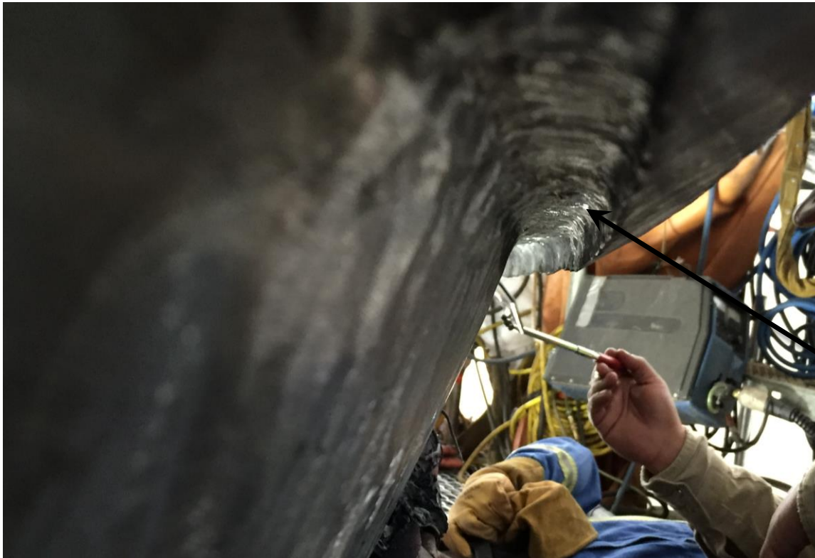
Knuckle Radius Bottom of Weld Deposit
