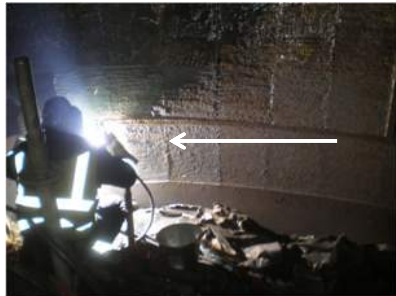
Gouging in process 2 – 3 mm material removed
