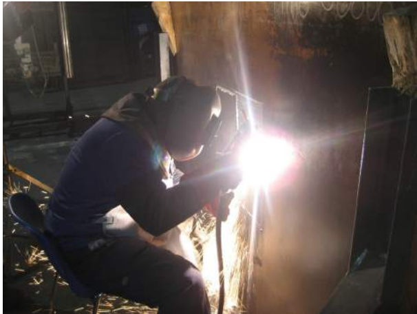
Removal of bonded cladding
