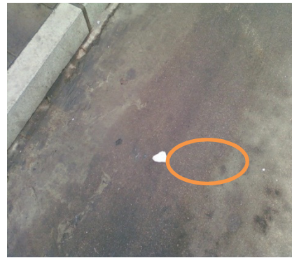
Solid material carried out by clean flue gas
