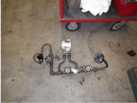
Fig. 5 : DP Assembly Removed (Left) and Impulse Lines Blocked (Right)
